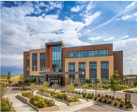
Dry Creek Medical Campus 145 Inverness Dr E Englewood, CO
