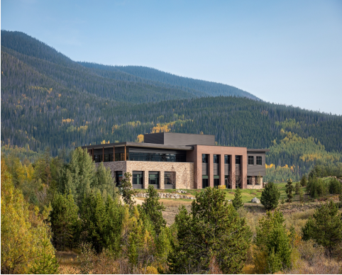
School Road Medical Center 68 School Road Frisco, CO
